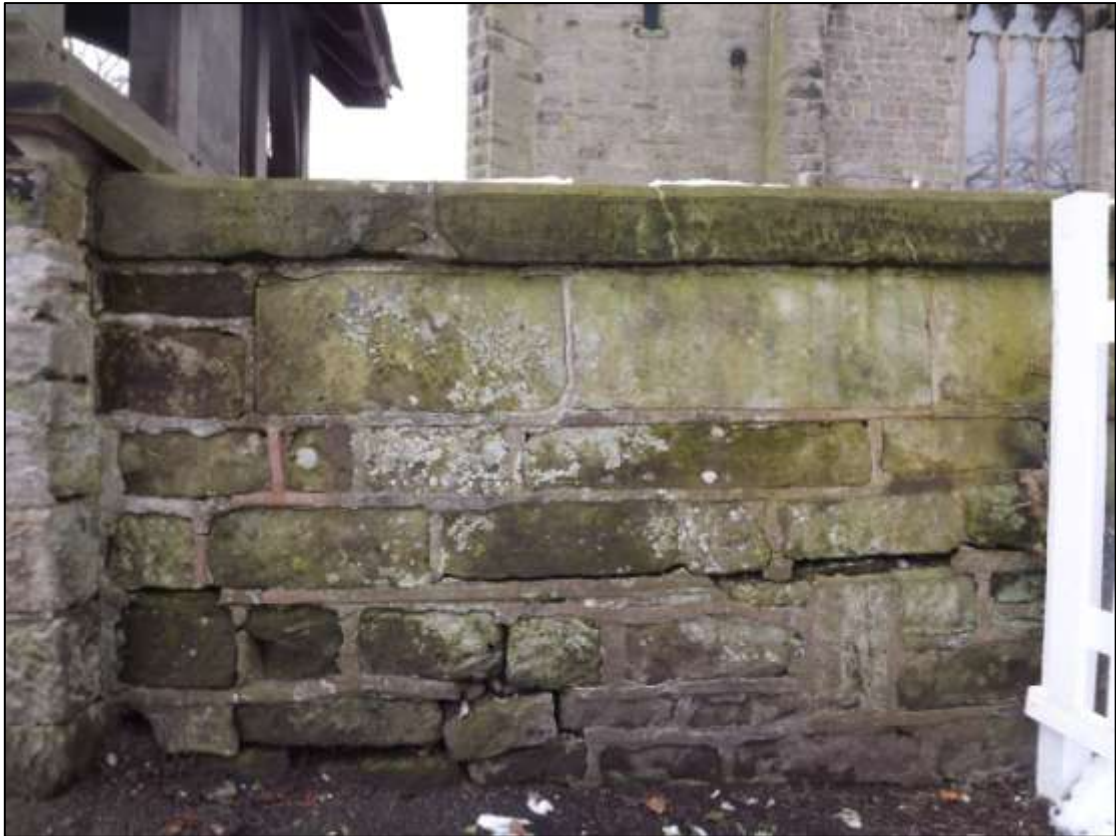
Figure 50 Churchyard boundary wall
