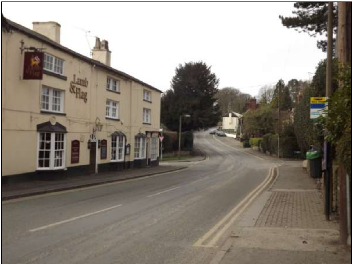
Figure 57 Haphazard paving surfaces
