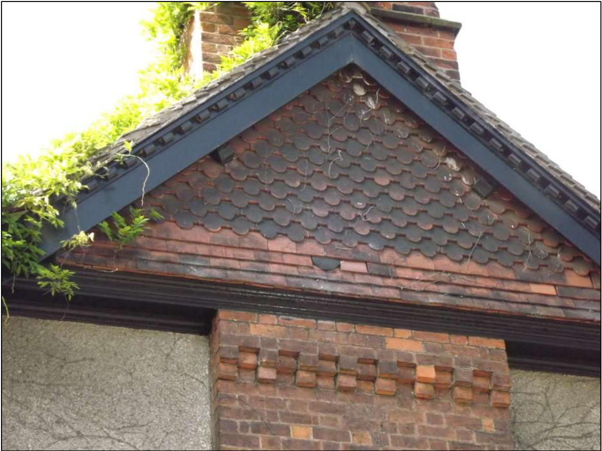
Figure 13 Roof detailing at Trubshaw House
