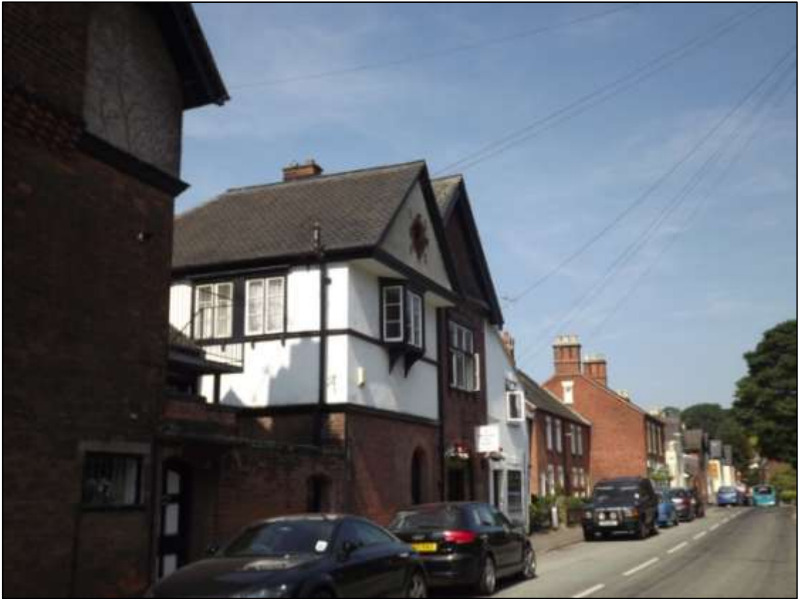
Figure 14 Roof detailing at Jasmine Cottage and Poacher's Cottage
