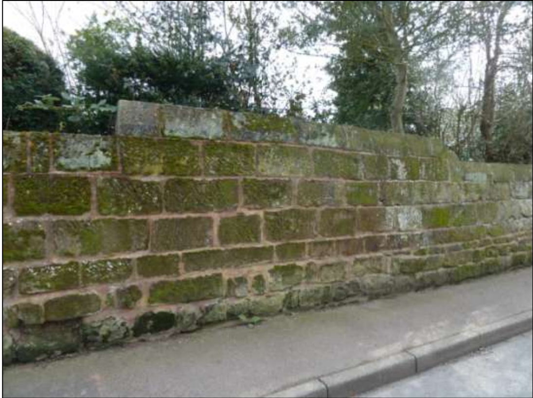
Figure 23 Boundary walls at Cherry Orchard House
