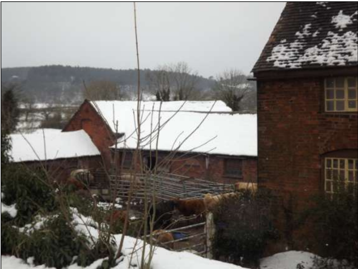
Figure 46 Church Farm and Barns
