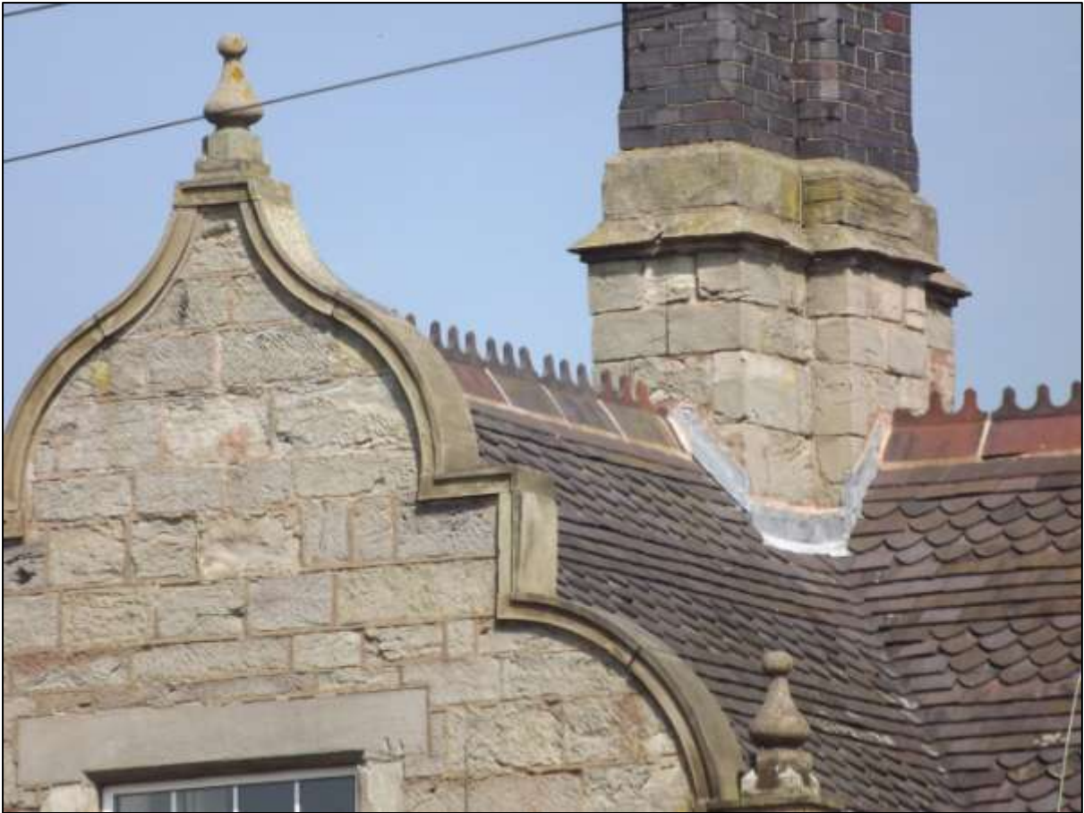
Figure 36 Roof detailing at Station House, employing fish scale tiles, Dutch gables and decorative ridge tiles
