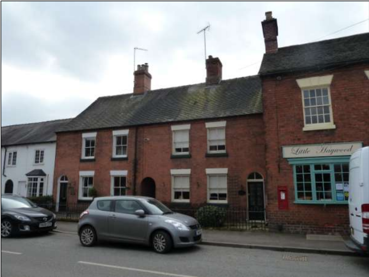
Figure 12 Main Road. The houses gradually step down in height
