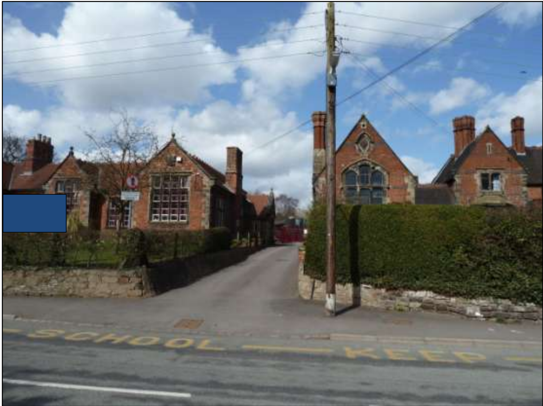
Figure 40 Primary School and School House
